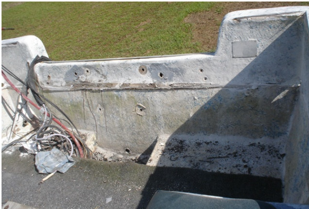
Figure 1 – Before the repair was commenced with the inner and outer skin being spongy. Rot occurred due to moisture accessing the ply core through the holes. Also note the compression around the holes.
